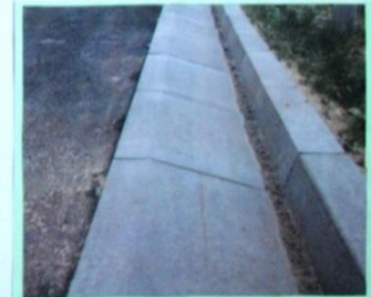
EXAMPLE OF OPEN SEWER
