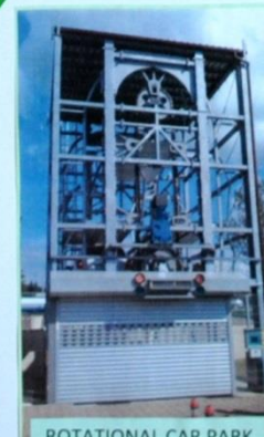
ROTATIONAL CAR PARK (CAPACITY 10 VEHICLES)
