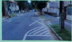
ROAD MARKING AT ACCESS
